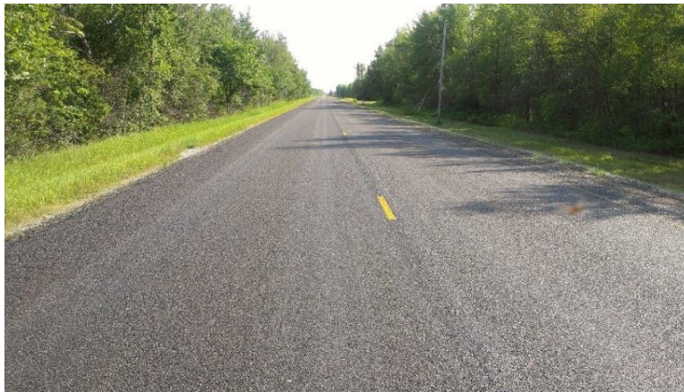
Figure 2 - TH 89 after placement of chip seal
